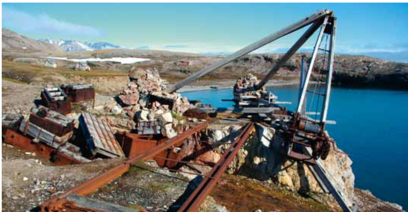
Marble Island. Crane brought to the English marble quarry in 1912.
