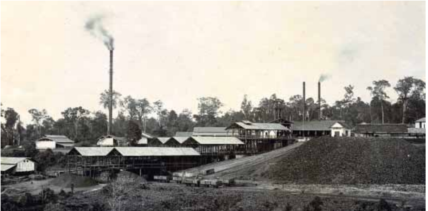
Shaft V and the sieving house of the Steenkolen Maatschappij Poeloe Laoet, on the island Poeloe Laoet, off the coast of Borneo. The mines were taken over by 'het Gouvernement' in 1913 and closed in 1931 (courtesy of Gerard de Graaf).
